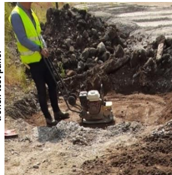
APEROFIN – Implementation of the trench test panel
