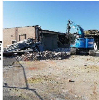
CIBER - Demolition of a commercial building
